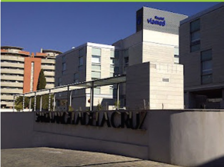
Hospital Viamed – Seville, Spain
